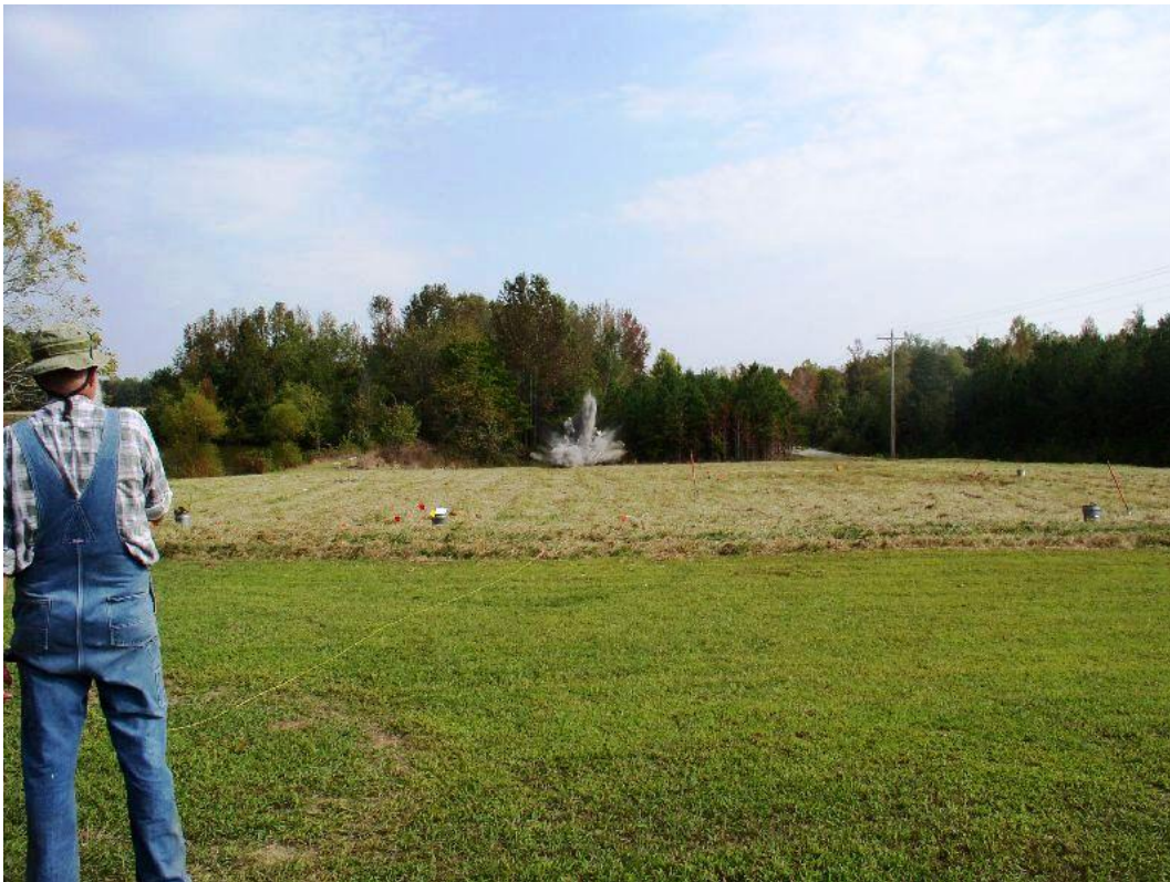
Figure C-18: Same demolition shot from firing line
