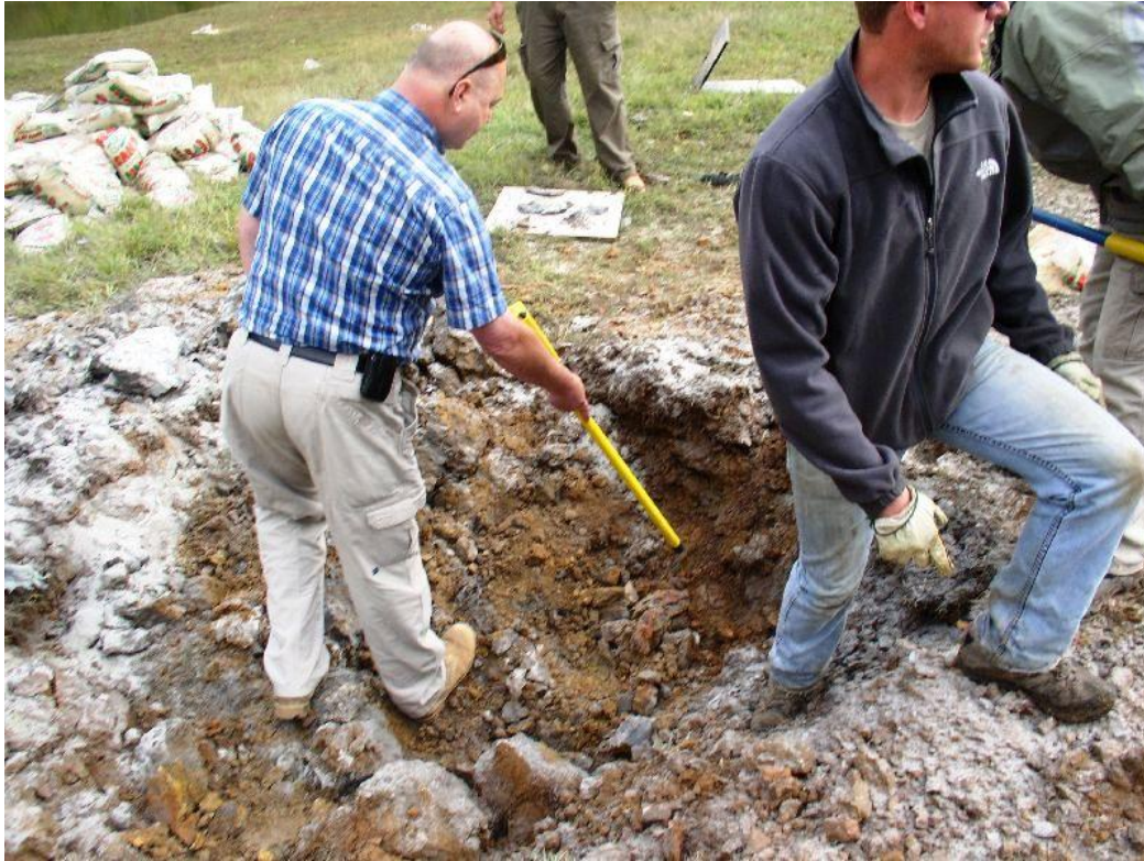
Figure C-27: USACE Safety Specialist clearing shot hole after detonation
