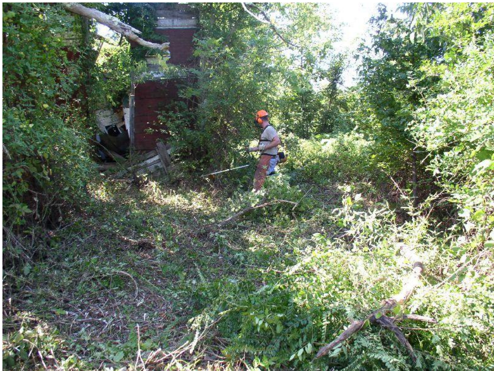
Figure C-8: Weedeater at work on Complex 2, Unit 5-2
