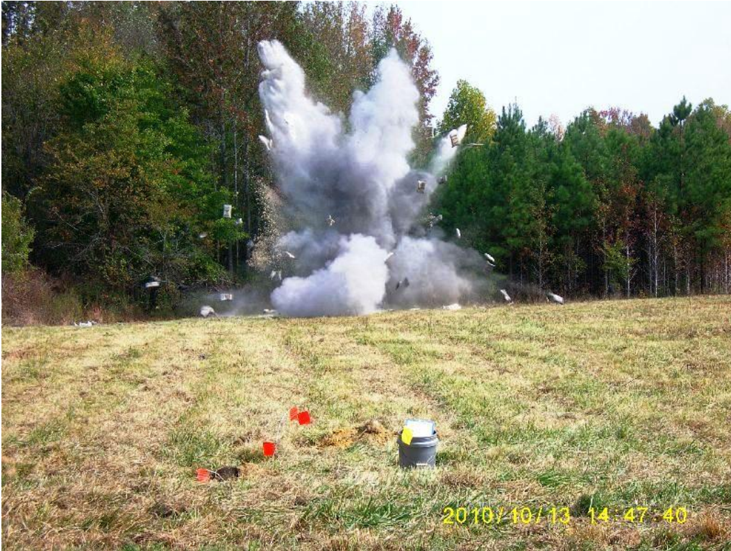
Figure C-17: Close-up of demolition shot showing sandbag scatter
